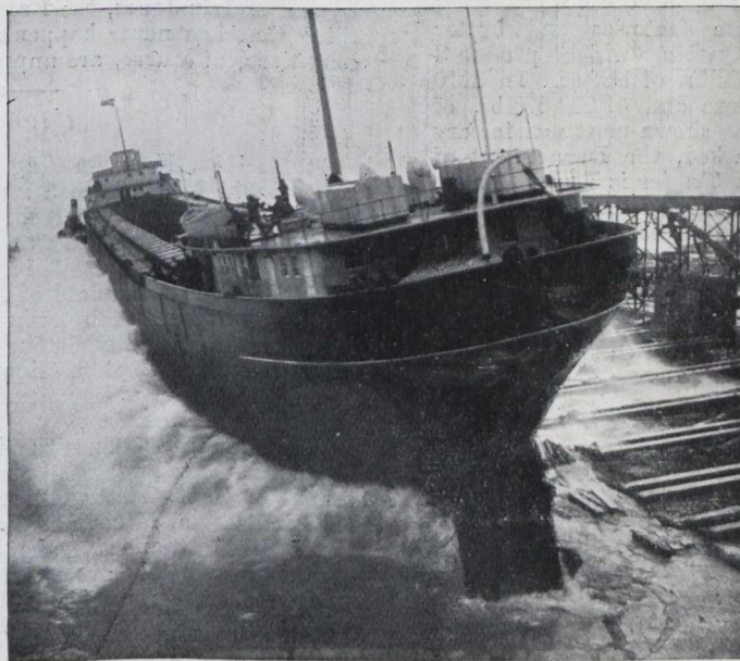
THE LAUNCH OF THE LAKE FREIGHTER, "W. GRANT MORDEN." Built by the Western Dry Dock and Shipbuilding Co., Port Arthur, for the Canada Steamship Lines, Ltd., and launched on April 4, 1914. She is 625 feet long, carries 85,000 bushels of wheat and made her first trip on May 9.
