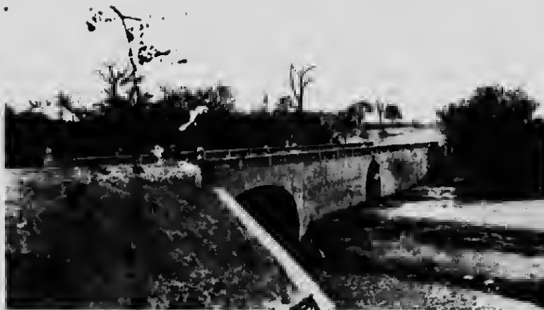
Concrete bridge on the Lake Shore Road crossing, Rosehill Farm. This bridge has been built sufficiently large with a view of the Toronto to Hamilton permanent Highway being constructed over this route.
