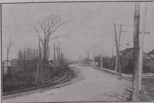
Dolarway Pavement, Lakeshore Road.
