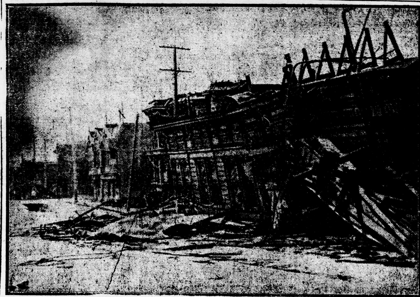
RUINS OF THE HOTEL VALENCIA AT SAN FRANCISCO. This Building, an Eight-Story Edifice, Collapsed with the First Shock. Forty Dead Bodies Have Been Taken from the Debris.
