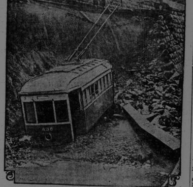
Tokyo no sooner recovers from an earthquake than it is hit by a disastrous flood, which makes 2,000 homeless. This trolley car crashed down an embankment when a supporting wall was undermined by the flood. Five persons were seriously injured.
