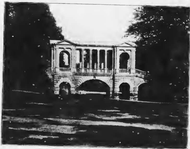
166.—THE BRIDGE, WILTON HOUSE.
