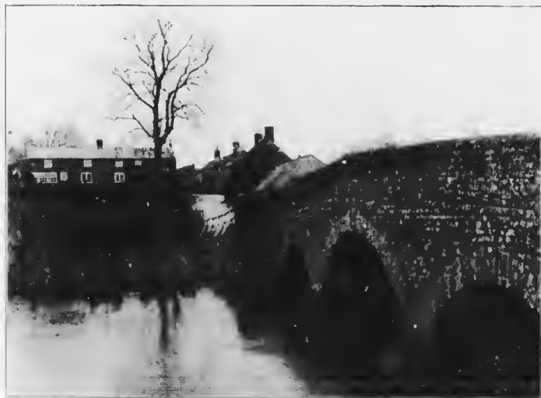
67. THE BRIDGE AND RIVERSIDE HOUSE, LOWER BOCKHAMPTON.
