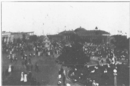
LOOKING OVER GRAND PLAZA TOWARDS MANUFACTURERS' BUILDING CANADIAN NATIONAL EXHIBITION
