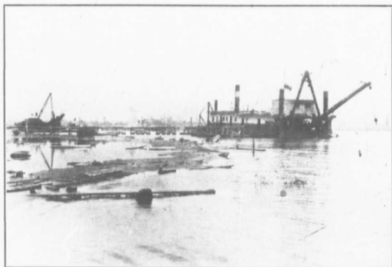
DREDGING THE LOCATION FOR A REVETMENT WALL AND DOCK SOUTH OF THE NEW WESTERN ENTRANCE TO TORONTO HARBOR
