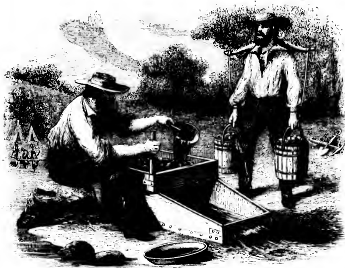
WORKING WITH THE ROCKER.
