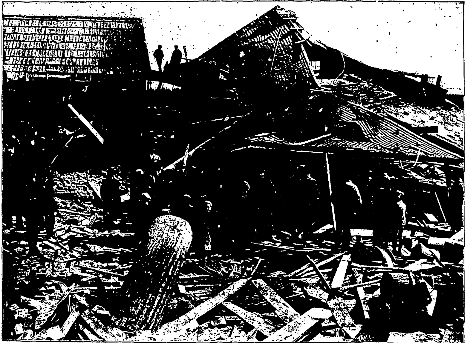
BOILER EXPLOSION AT RIDGETOWN, ONT.
