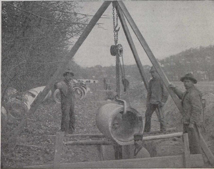
A Triples Block hung from a temporary rigging and used for laying pipe.
