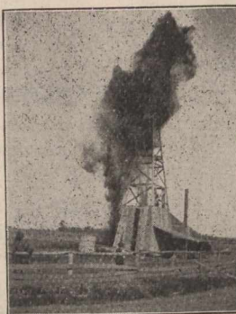
Torpedoeing an oil well at Petrolea, Ont
