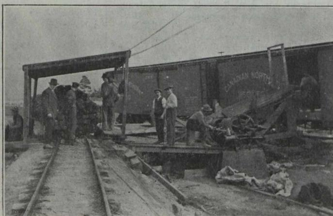
Fig. 5.—Loading Treated Ties into Box Cars.
