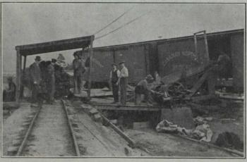
Fig. 5.-Loading Treated Ties into Box Cars.
