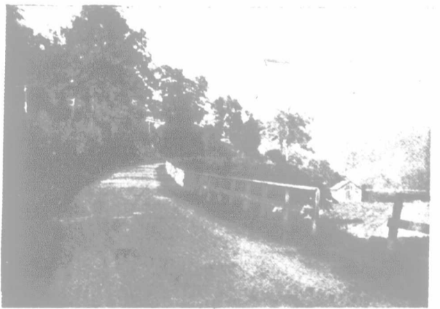
FIG. 2.—TYPE OF ROAD AFTER IMPROVEMENT.
