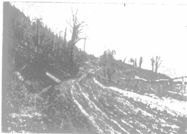
FIG. 1.—TYPE OF ROAD BEFORE IMPROVEMENT.
