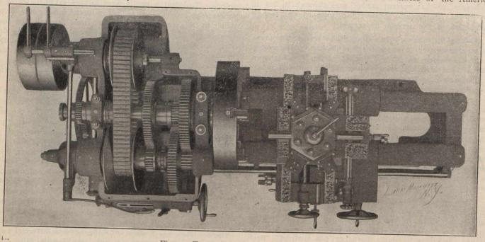
Fig. 2.—Turret Lathe without Gear Case.
