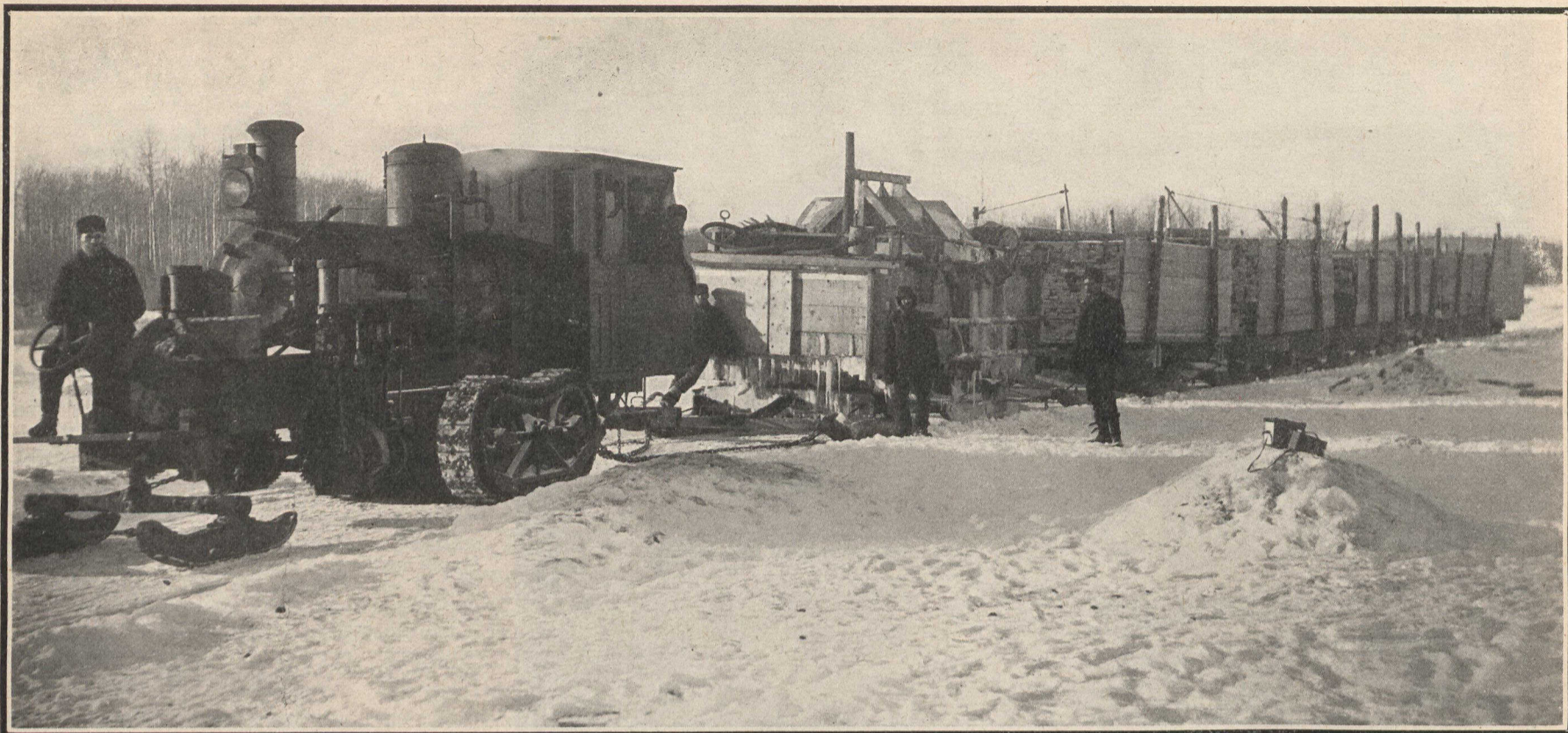
Sturgeon Lake Lumber Company's Snow Locomotive Hauling 100,000 feet of Lumber from the Mill to Prince Albert, Sask., a distance of Thirty-five Miles
