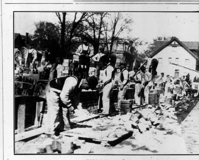
WITH THE BUILDERS. Masons at work on foundations of a large apartment house, which will be erected on Jarvis-street.
