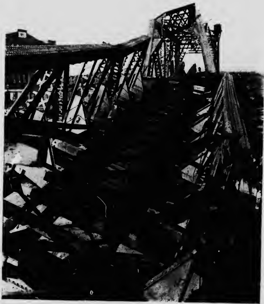
Destroyed railroad bridge, Eastern war zone.
