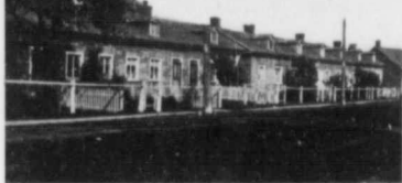
Cottages at Valleyfield.
