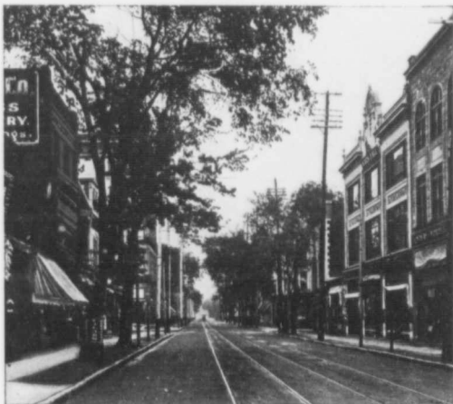
St. Catherine Street, near Peel. (5 30 A.M.)
