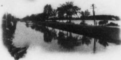
Some Views along the Banks of the Chambly Canal, near St. Johns.
