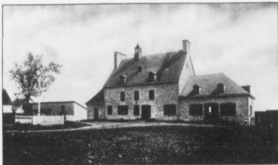
St. Gabriel Farm-house on the river bank, Point St. Charles (owned by the Congrégation de Notre Dame). Erected 1662.
