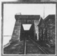
Victoria Tabular Bridge, showing construction of present Bridge.
