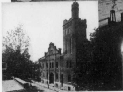
Drill-Hall and Victoria Rifles' Armoury.
