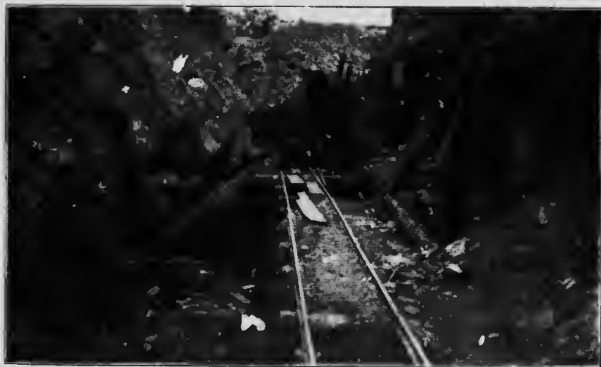
Dumping ore from open cut into chute, through apraise from lower level, Lone Star mine.
