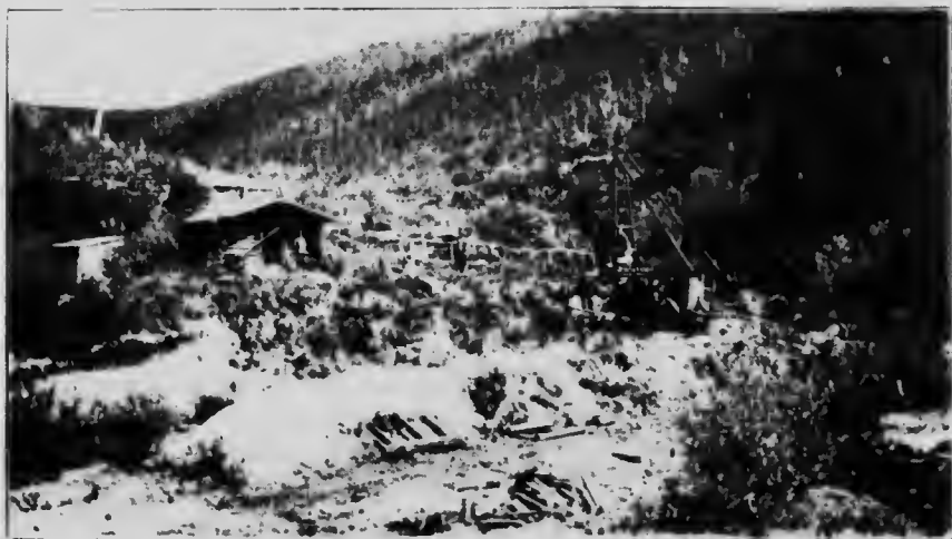
Discovery Pup, looking in a N.W. direction up the pup from Bear creek. Keystone drill, in the foreground, is testing the gravels on the right limit of the creek.
