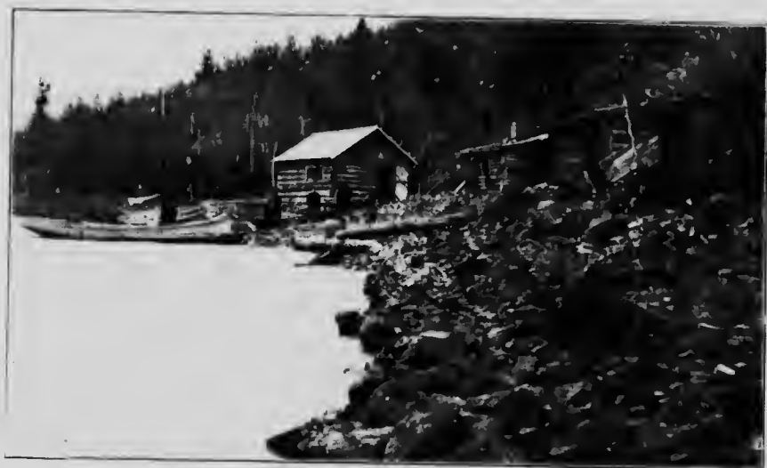
Buildings of Dail and Fleming, on the Humber group, shore of Windy Arm.
