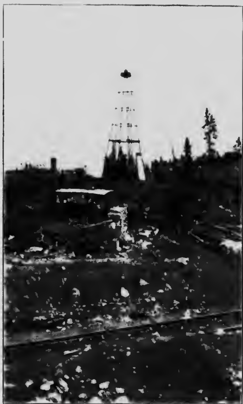
Shot drill at work on the Best Chance copper prospect, Whitehorse district, Y.T.
