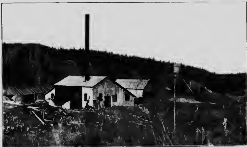
Power-house, store, shaft-house, forge, etc., the Pueblo copper mine, Whitehorse, Y.T.
