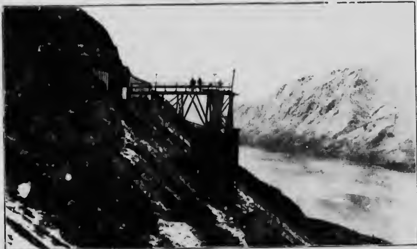
Track at main entry, chute, and ore pocket, Venus mine. When in operation the ore is conveyed from this pocket by aerial gravity tram to the mill, which is located on the shore of Windy Arm, about 1,100 feet below.
