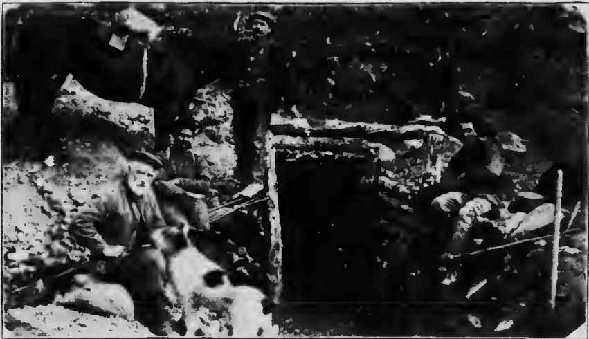
Tunnel entry, the Olive mineral claim.
