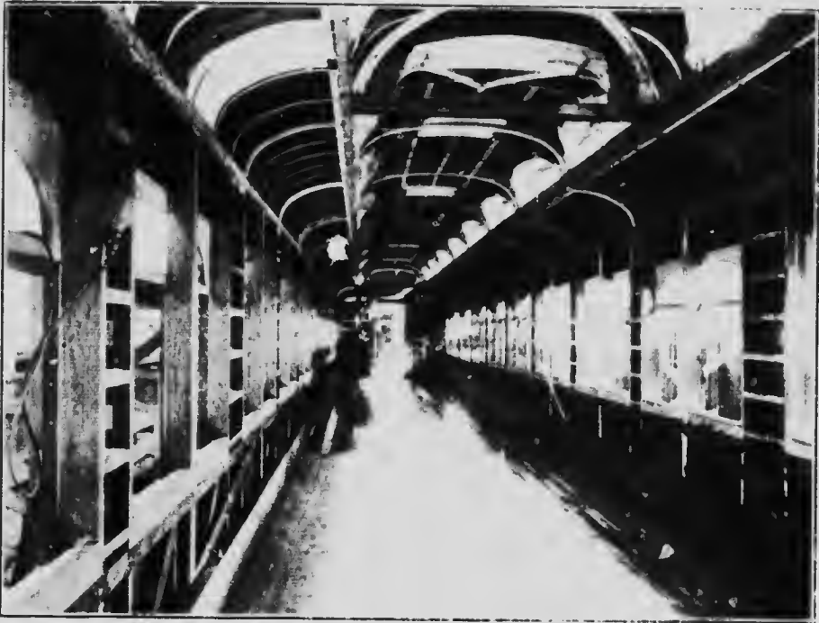
COURTESY CANADIAN CAR & FOUNDRY CO. Interior of Unfinished Passenger Coach—Curplings of Birch and AS; Floor of Maple; Structures of Hard Pine Truss Planks of Hard Pine; Sash of Mahogany.
