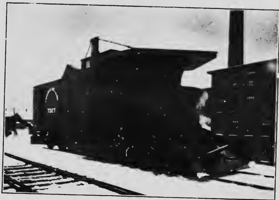
(COURTESY CANADIAN CAR & FOUNDRY CO.) Finished Snowplough: Sheeting of Hard Pine. Canadian Car & Foundry Co., Ltd., Amherst, N.S.
