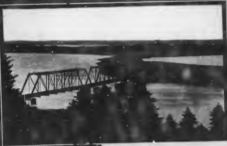
Hortonville Railway Bridge, Gaspereaux River.
