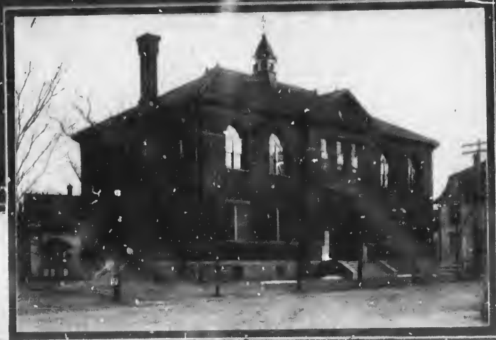
Court House, Kentville.
