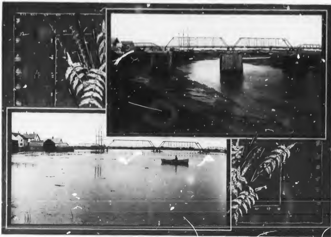
Bridge at Port Williams.
