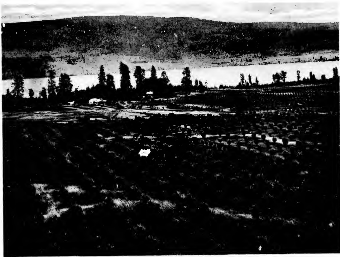
SHORT'S POINT, DUNSMUIR ESTATE, OKANAGAN LAKE, B.C.
