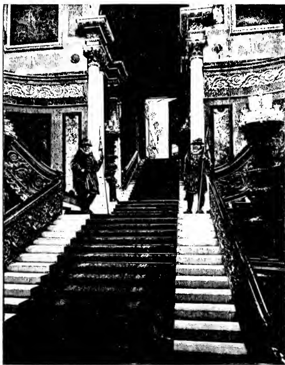
Buckingham Staircase. Escalier de Buckingham.
