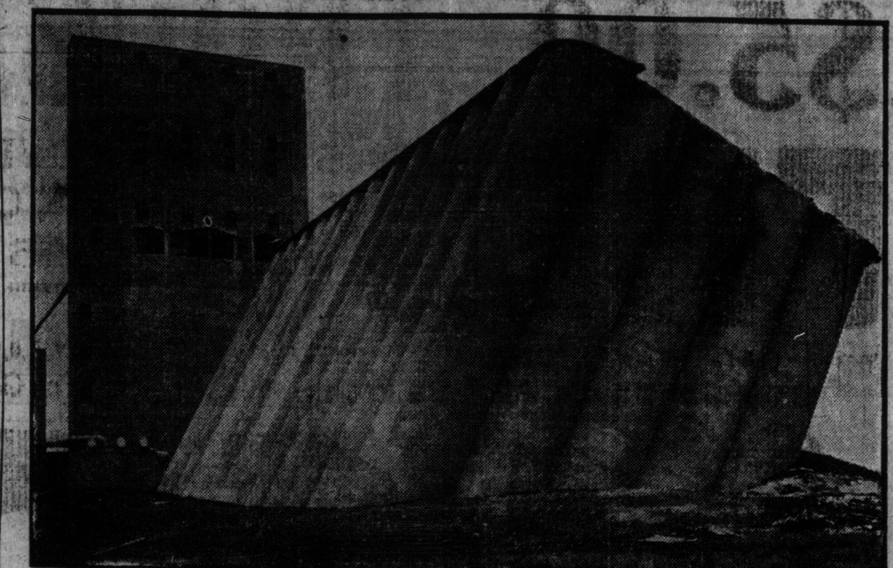
Tilting of the huge C.P.R. terminal elevator at the Transcona yards, Winnipeg, on Saturday last. The elevator still contains one million bushels of wheat.
