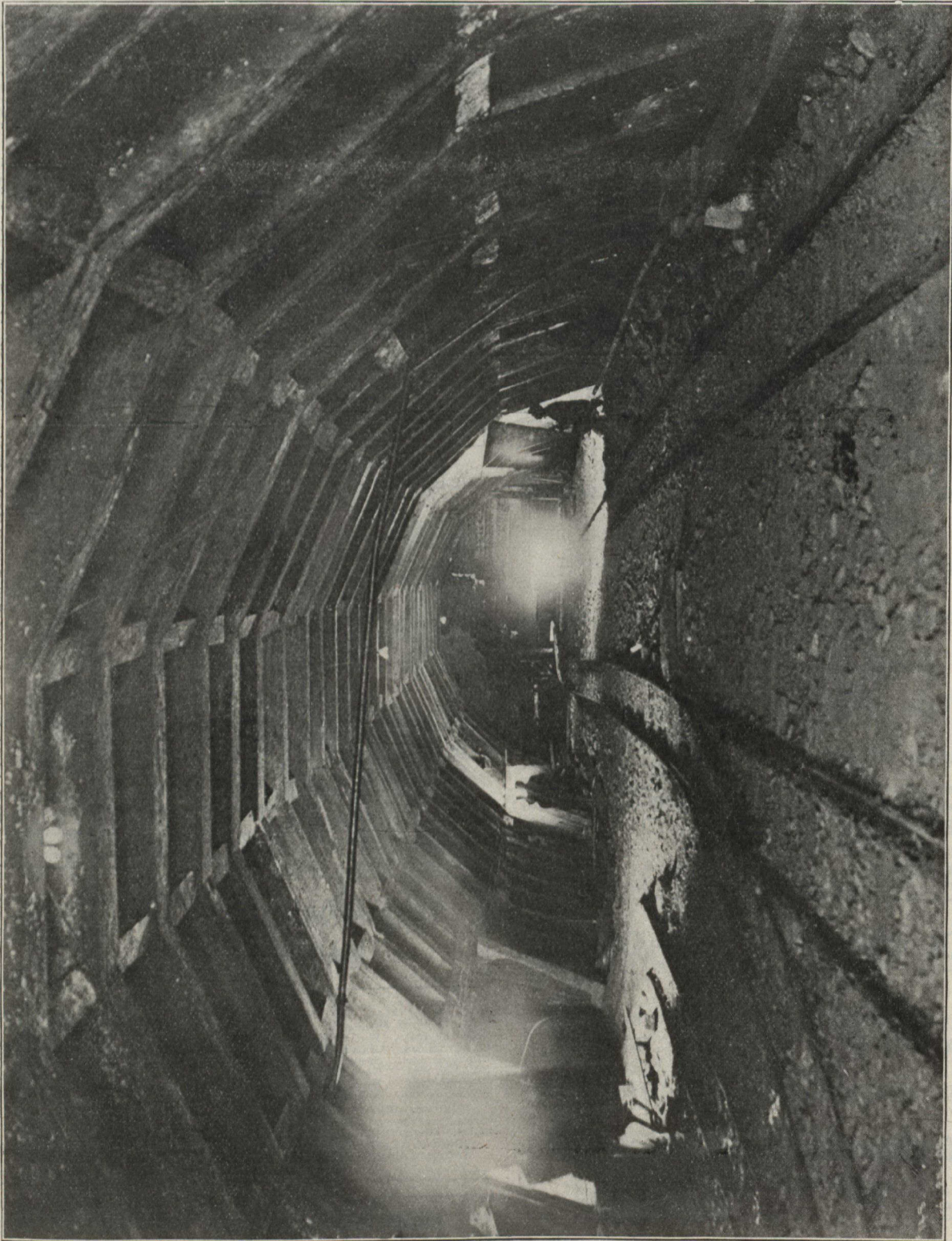
Flash Light Photograph of the Tunnel under Niagara River. The end is boarded up to keep out the spray from the Falls, which hindered the workmen.
