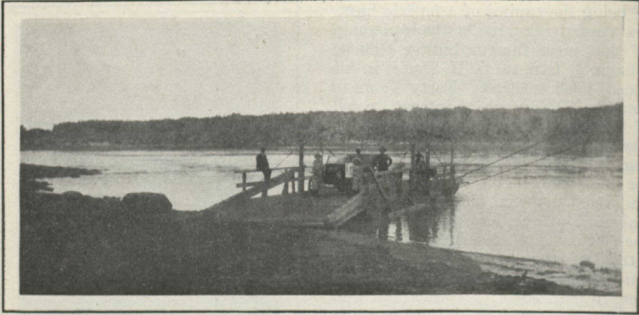
THE FERRY AT BATOCHÉ Propelled by the current of the River
