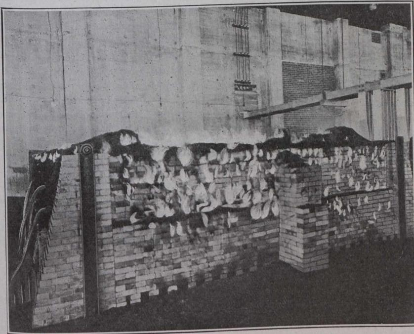
Fig. 3.—Electric Furnace for Manufacturing Crystolon.
