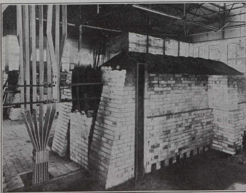
Fig. 2.—Electric Furnaces for Manufacturing Crystolon.
