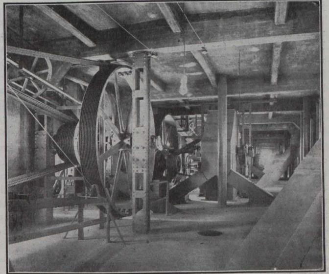
Fig. 9.—View of Top Floor Showing Elevator Heads and Drive.
