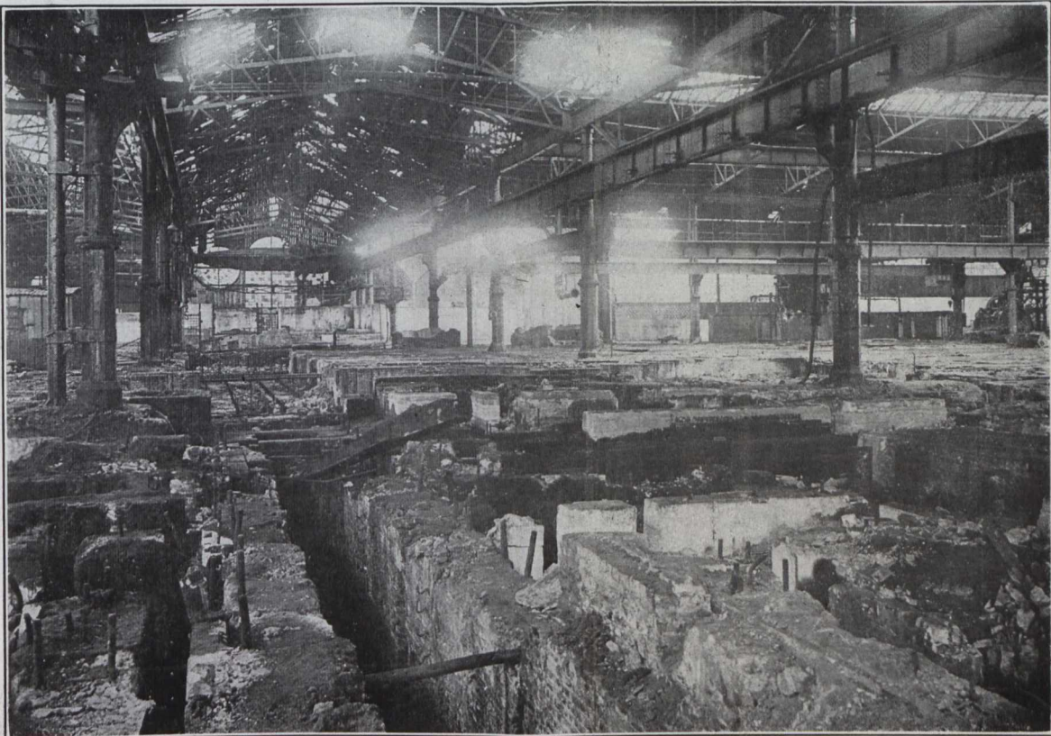
Rolling-Mill of the Longwy Steel-Plant.
