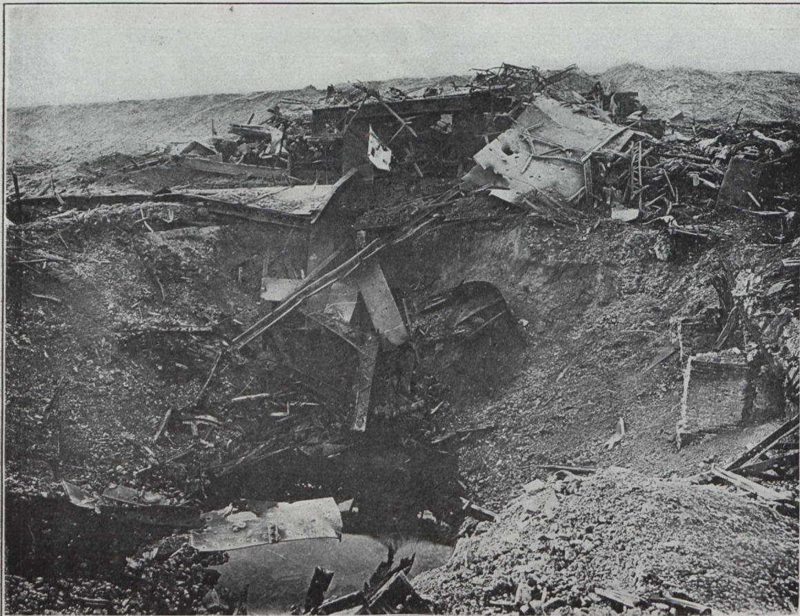
Shaft and Plant at Bethune.
