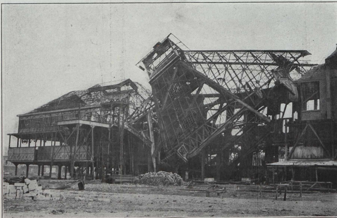
Surface Plant at the No. 4 Shaft, at Courriere.
