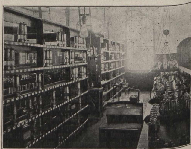
Interior of Lamp House.
