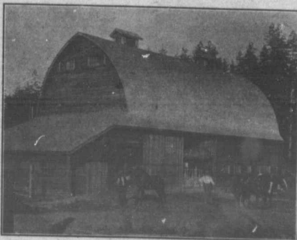
A Fine B.C. Dairy Barn as it Appears Completed
