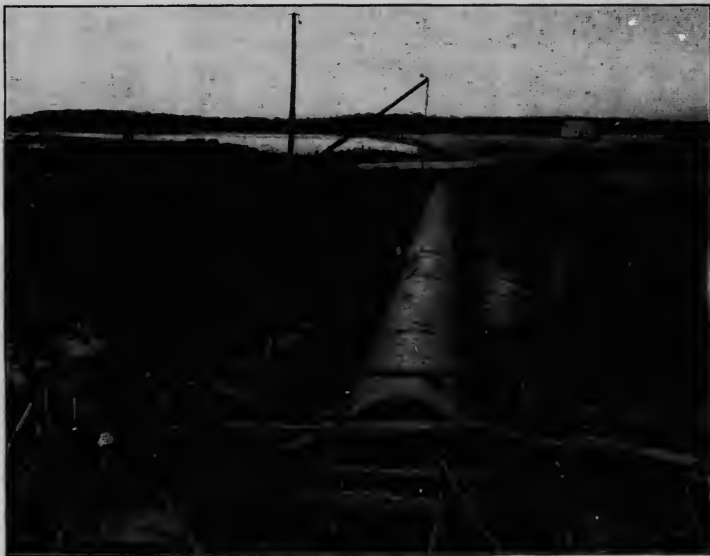
FIG. 6. VIEW OF SINGLE-PIPE CULVERT FOR GREASE RIVER DURING CONSTRUCTION; SOULANGES CANAL WORKS, CANADA.
