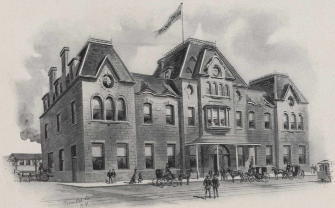
West End Railway Passenger Station.
