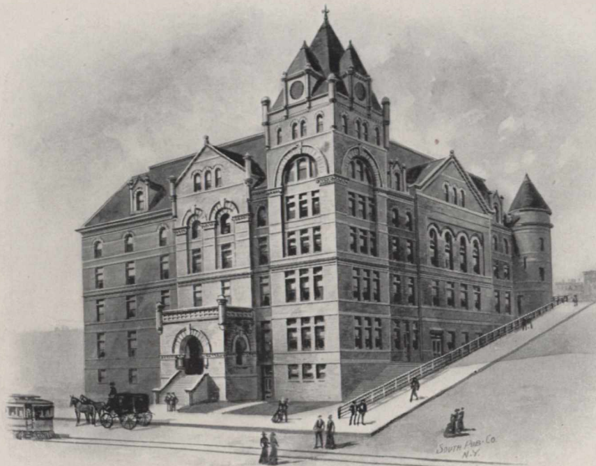
New Court House. Water Street Elevation. Stone for this building furnished by W. G. Ellis, from Petites Quarries. Woodwork for this building executed by Horwood Lumber Company, Limited.
