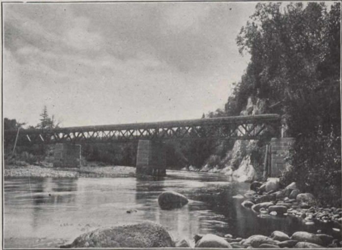
Newfoundland Railway Bridge.
