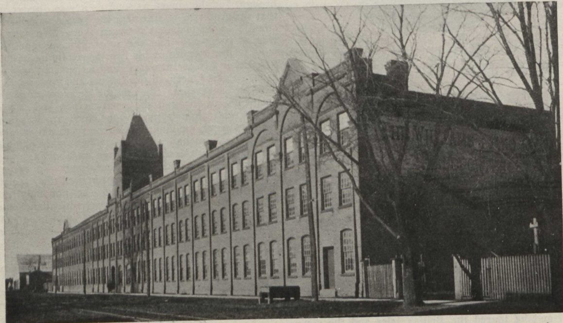
Oshawa—The Williams Piano Company's Factory is a Well-built Structure, Indicating Prosperity and Enterprise.
