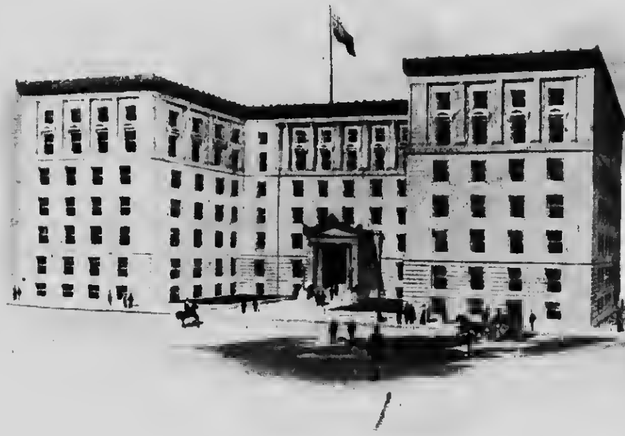
Edifice du "Board of Trade"
