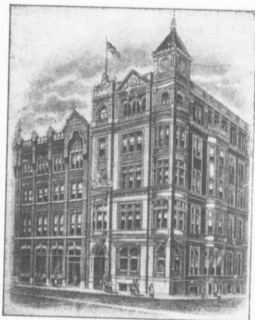
HEAD OFFICE BUILDING, MONTREAL.
