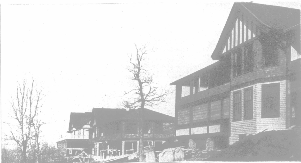
SANATORIUM AT NINETTE. EAST VIEW.
