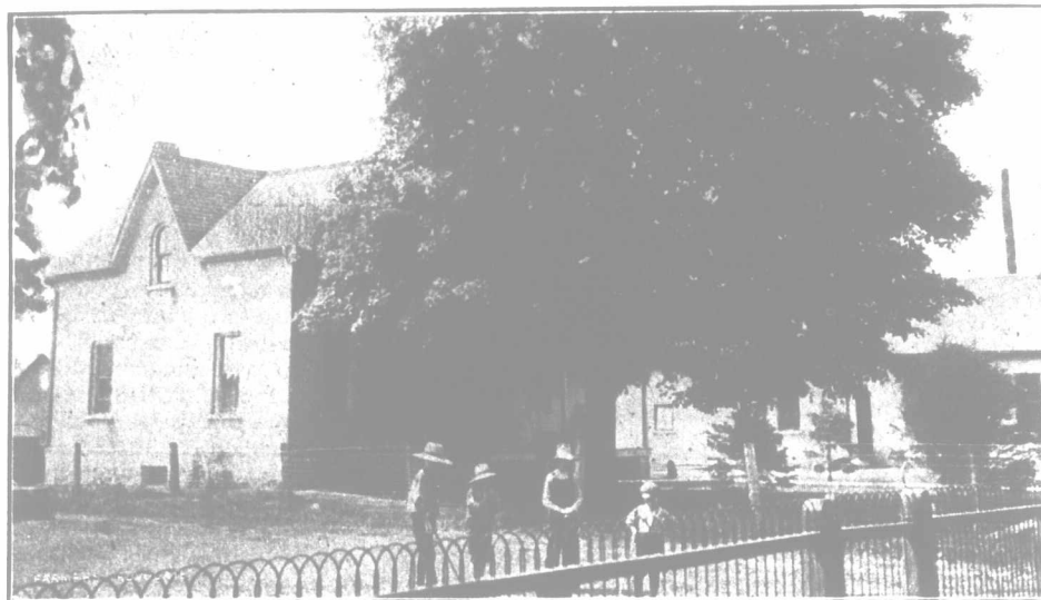
Maker's Residence at Bright Factory.
