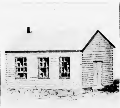
LOG CHURCH, BUILT 1847.
