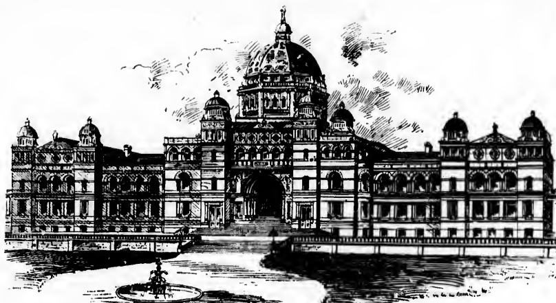
LEGISLATIVE BUILDINGS, BRITISH COLUMBIA (Under Construction).
