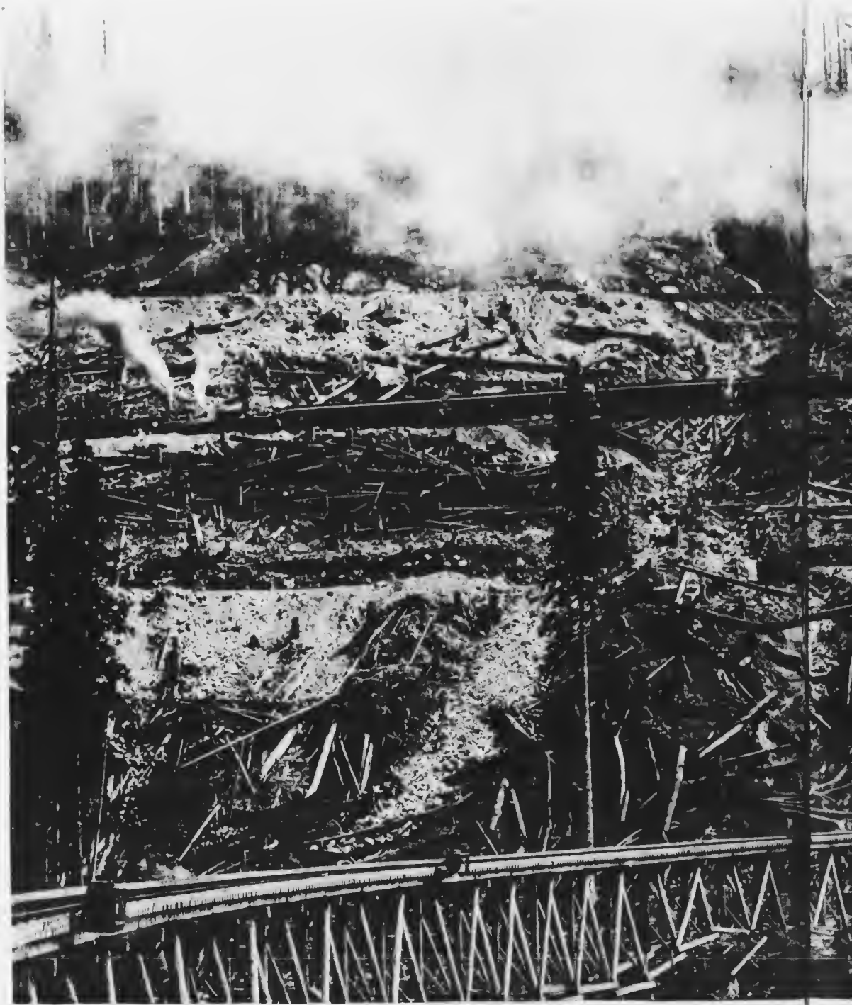
THE "ZIG-ZAG" WHEREBY THE CASCADE MOUNTAINS WERE NEGOTIATED The Great Northern Limited, of seven Pullmans, weighing 280 tons, had to be lifted over the steps of the temporary line was abandoned
