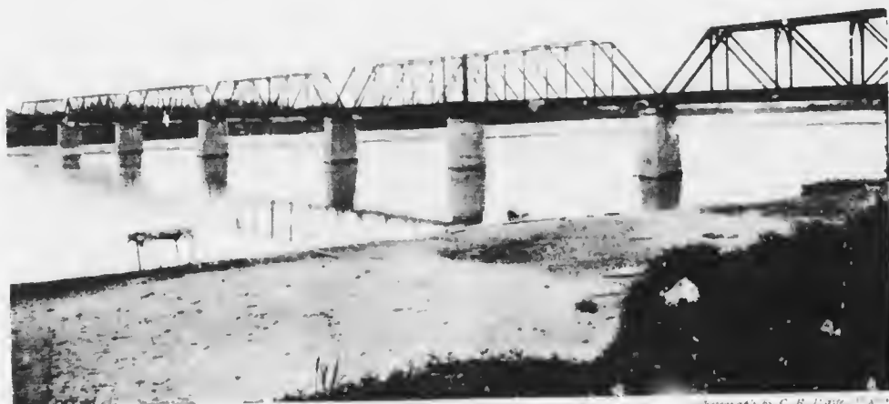
BRIDGE OVER THE PAPALOAPAM RIVER, ON THE VERA CRUZ AND ISTHMUS RAILWAY The total length is 1,100 feet.
