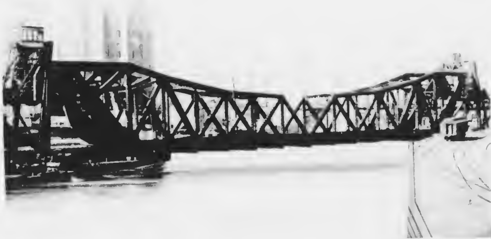
275-FOOT DOUBLE-LEAF DOUBLE-TRACK SCHERZER ROLLING LIFT BRIDGE ACROSS THE CHICAGO RIVER AT THE ENTRANCE TO THE GRAND CENTRAL STATION, CHICAGO.
