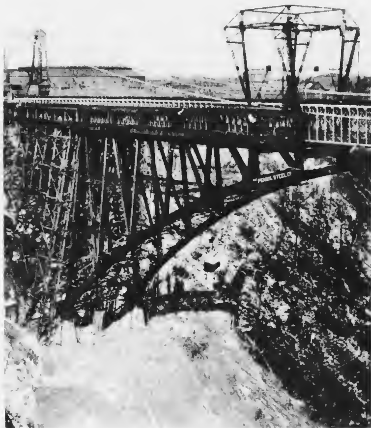
BUILDING THE SINGLE SPAN STEEL ARCH BRIDGE AROUND THE OLD SUSPENSION BRIDGE ACROSS NIAGARA'S GORGE
