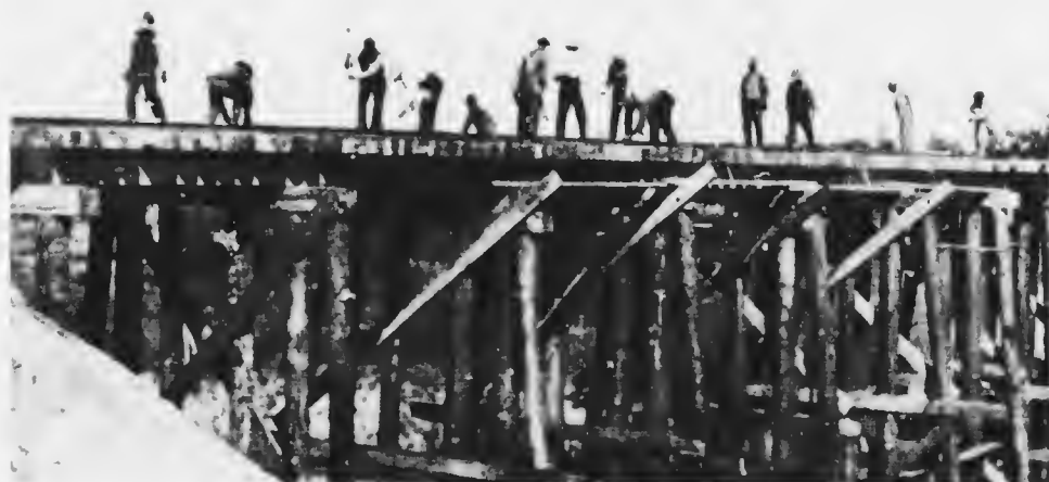
BUILDING A TEMPORARY TREESTLE BRIDGE IN NORTH SASKATCHEWAN.
