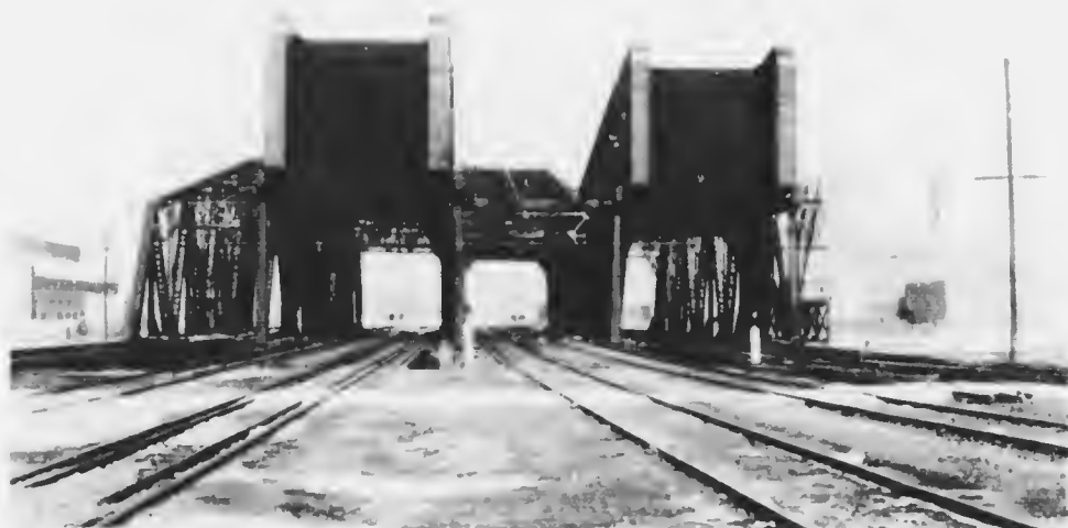
FOUR SINGLE LEAF DOUBLE TRACK SCHIRZER ROLLING LIFT BRIDGES, SIDE BY SIDE, FORMING AN EIGHT-TRACK STRUCTURE ACROSS THE SHIP CANAL, CHICAGO.
