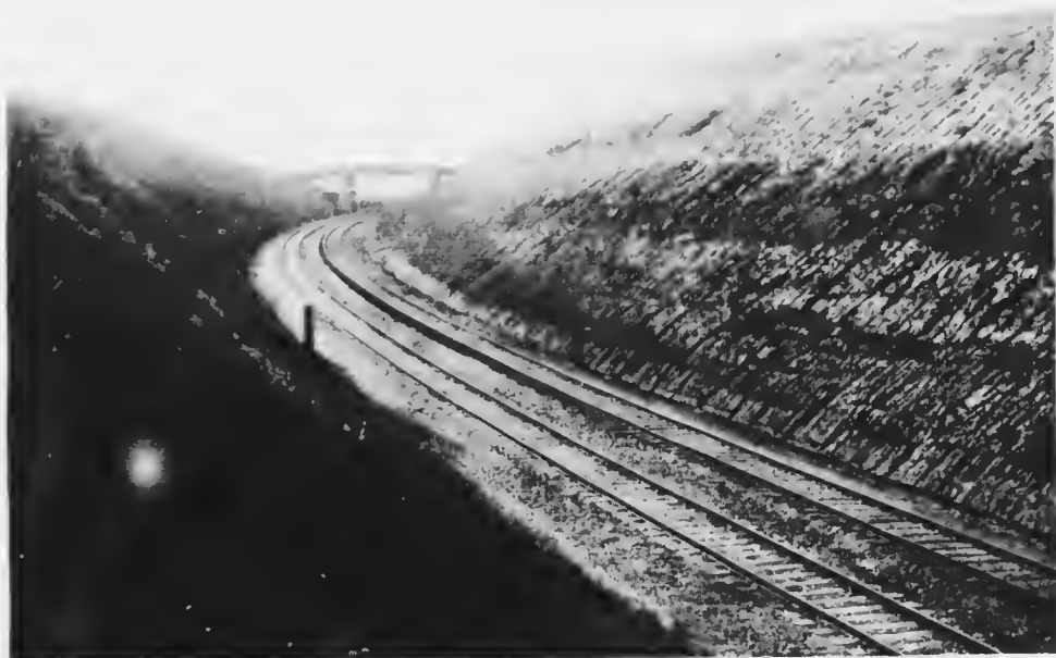
THE BIG CUTTING ON THE LANE CUT-OFF
