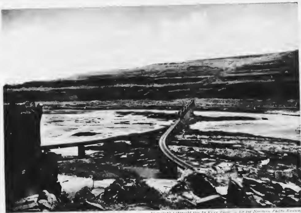
Photograph Copyright 1904 by River Falls for the Northern Pacific Railway. THE CELILO BRIDGE CROSSING THE FALLS OF THAT NAME UPON THE COLUMBIA RIVER TO ENABLE THE OREGON TRUNK LINE TO ESTABLISH A CONNECTION WITH THE NORTH BANK ROAD. On the north side of the waterway the bridge has a V approach.
