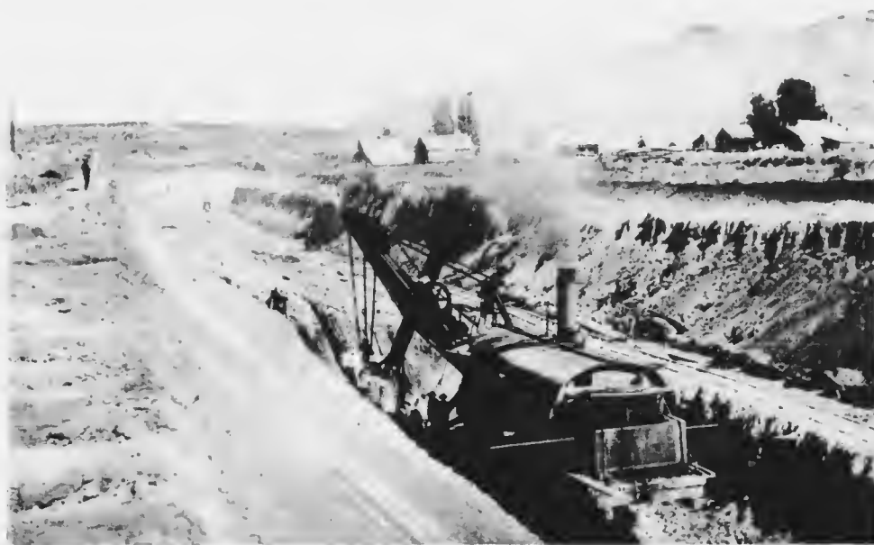
STEAM SHOVEL EXCAVATING THE BOTTOM LEFT OF THE BECKWOURTH TUNNEL APPROACH, THE SUMMIT LEVEL OF THE WESTERN PACIFIC RAILWAY, 4,956 FEET ABOVE THE SEA.
