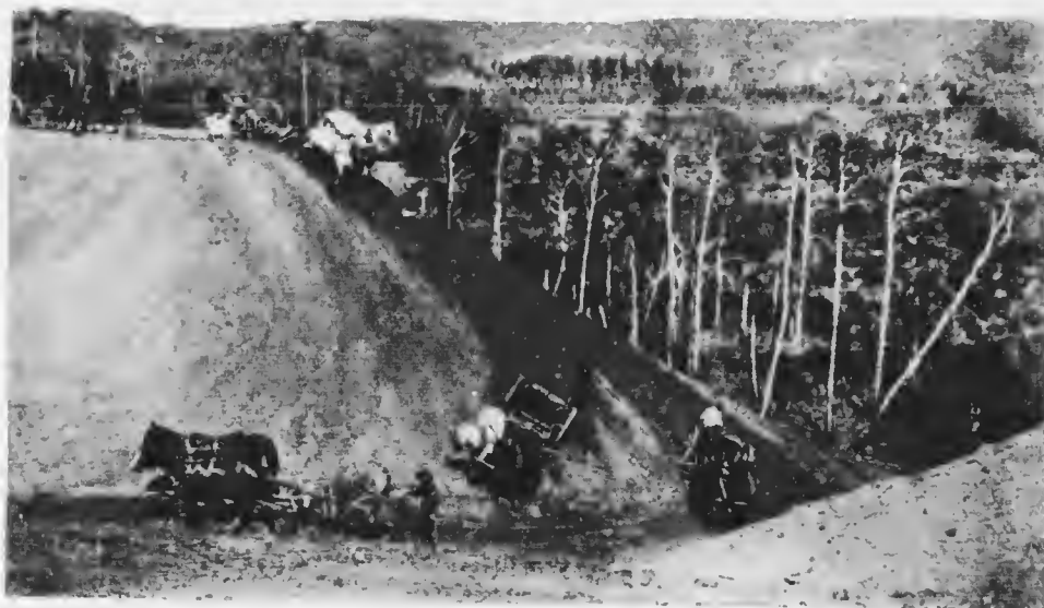
BUILDING A HIGH EMBANKMENT.
