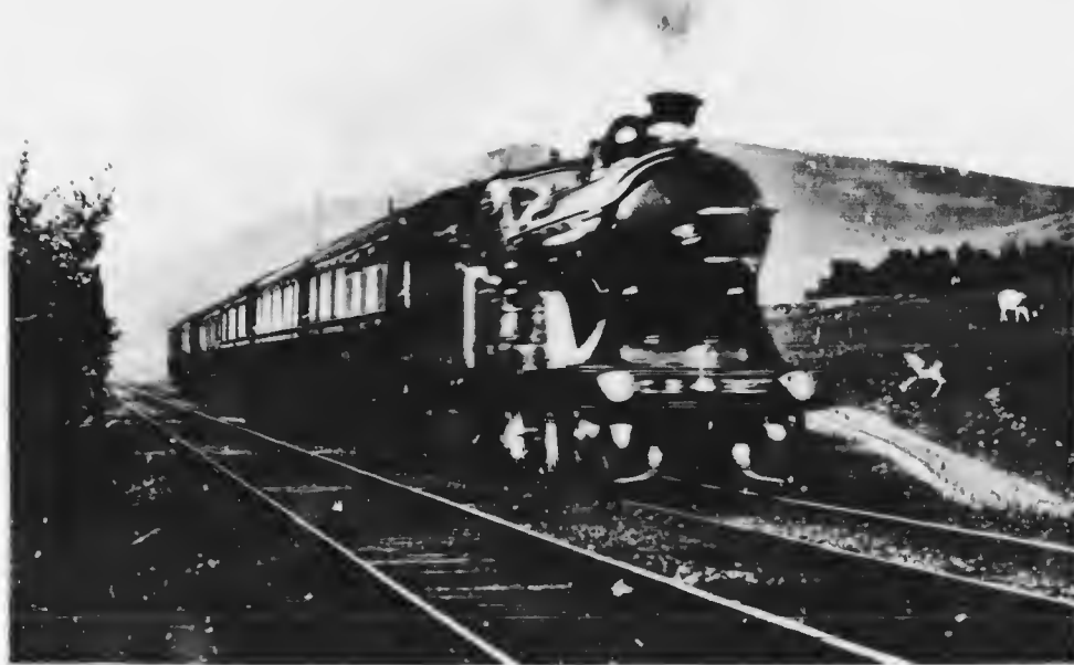
THE 2 P.M. GLASGOW-CARLISLE EXPRESS AT ABINGDON
