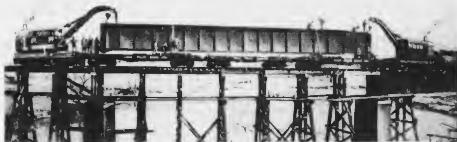
HOW WRECKING CRANES LOWER INTO POSITION A MASSIVE PLATE GIRDER
