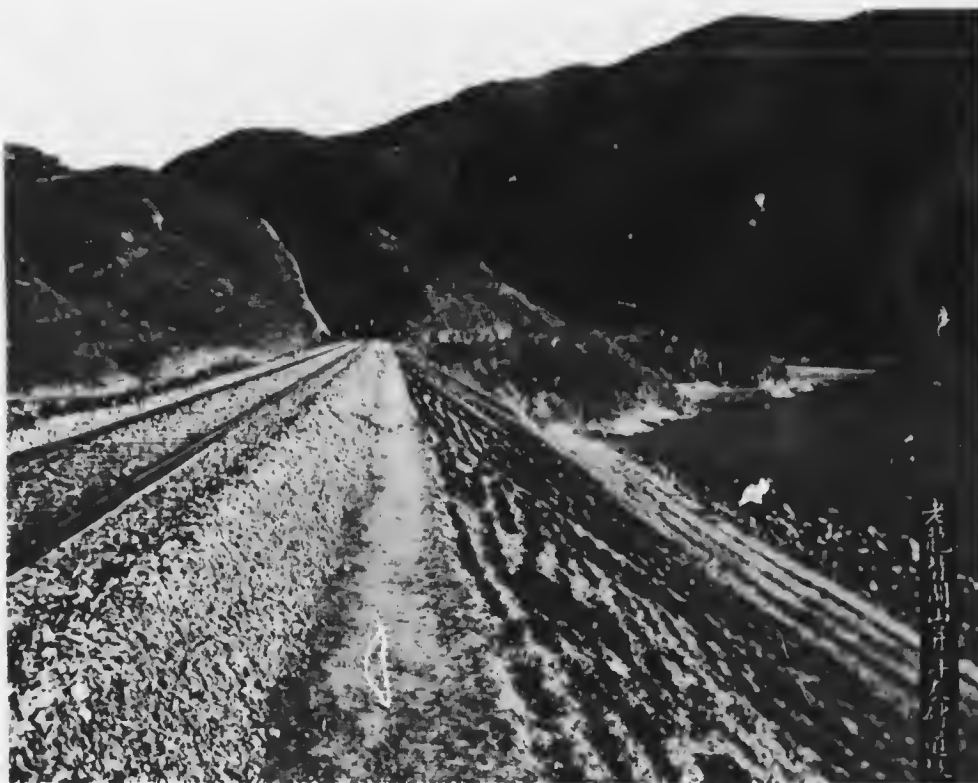
A TYPICAL STRETCH OF TRACK AMONG THE MOUNTAINS ON THE PEKING-KALGAN RAILWAY, SHOWING SOLID CUT OF THE GRADE.
