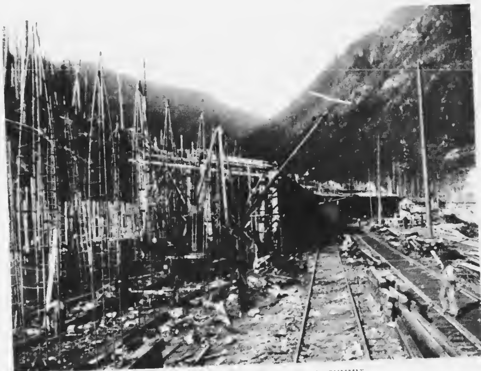
NEW CONCRETE SNOW-SHED, CASCADE SUMMIT. The ferro-concrete sheds in course of construction. This photograph conveys a graphic idea of the steepness of the mountain sides.
