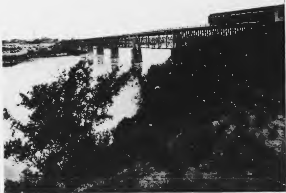
LAREDO BRIDGE, BETWEEN LAREDO, TEXAS, U.S.A., AND NUEVA LAREDO, MEXICO It comprises six spans each of 175 feet, with an approach at each end 65 feet in length.
