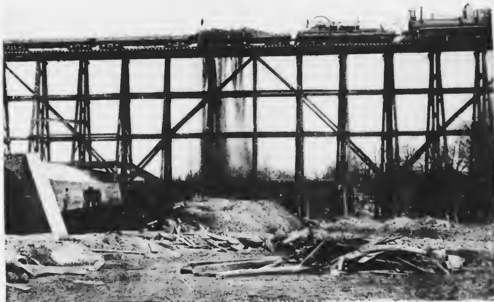
THE LIDGERWOOD UNLOADER DISCHARGING MATERIAL FOR AN EMBANKMENT TO REPLACE A TRESTLE.
