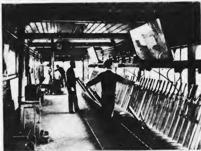
ST. PANCRAS JUNCTION SIGNAL BOX.
