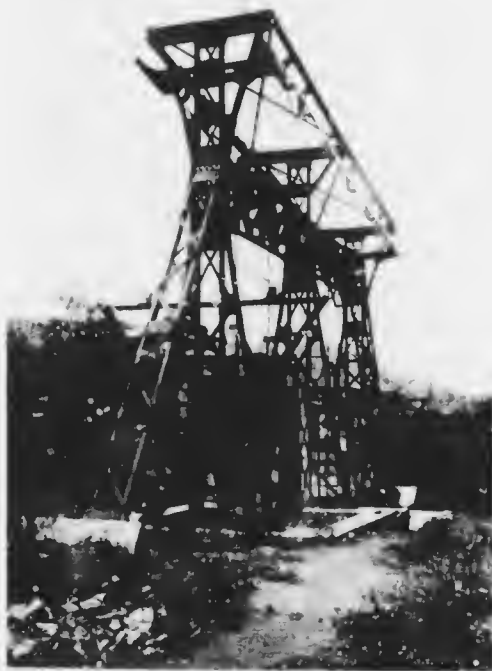
A TENSION STATION, SHOWING THE TOWERS WITH THE CONCRETE BLOCKS WHEREBY THE LINE IS KEPT TAUT
