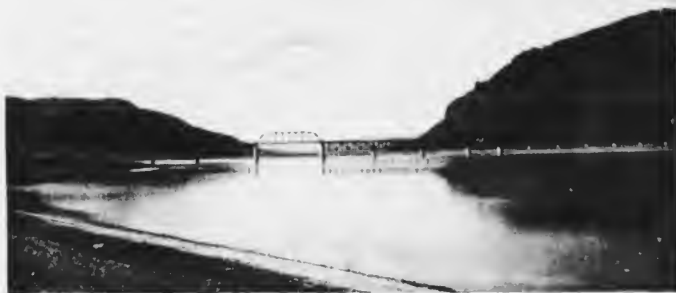
THE MASSIVE STEEL BRIDGE WHICH CARRIES THE CHICAGO, MILWAUKEE AND PUGET SOUND RAILWAY ACROSS THE COLUMBIA RIVER, NEAR BEVERLY, WASHINGTON. It is 2,740½ feet in length.
