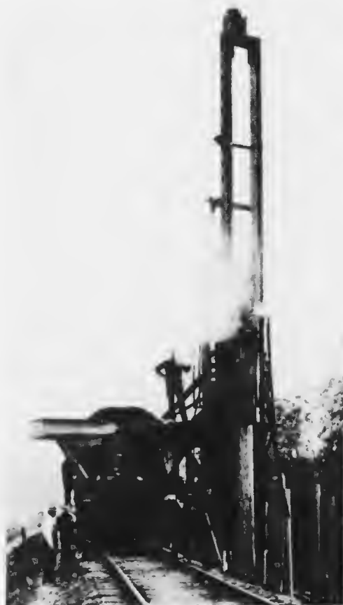
FRONT VIEW OF BUCYRUS PILE-DRIVER, SHOWING STEAM HAMMER AND SLEWING MOTION.
