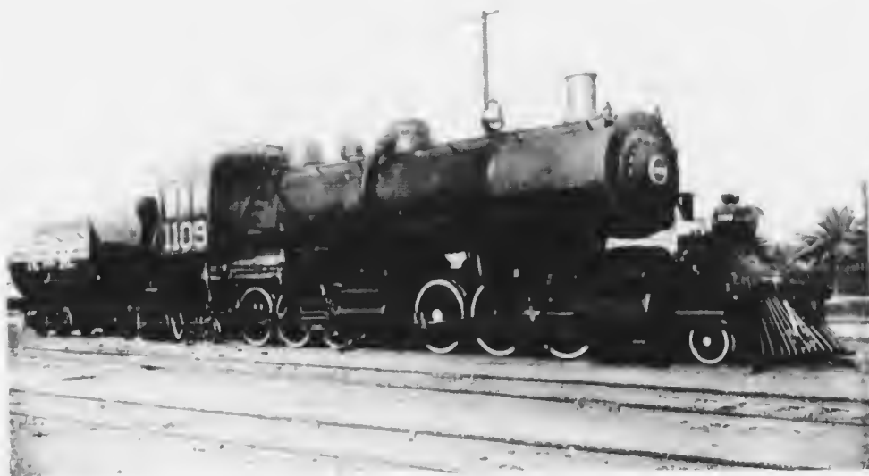
NATIONAL RAILWAYS OF MEXICO'S MAJESTIC ARTICULATED COMPOUND OIL-BURNING FREIGHT LOCOMOTIVE
