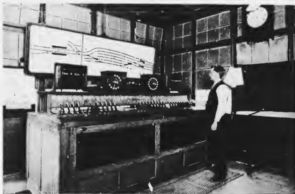
ONE OF THE SIGNAL BOXES AT WEST KENSINGTON JUNCTION ON THE METROPOLITAN DISTRICT RAILWAY, SHOWING LEVER FRAME AND ILLUMINATED TRACK DIAGRAM.
