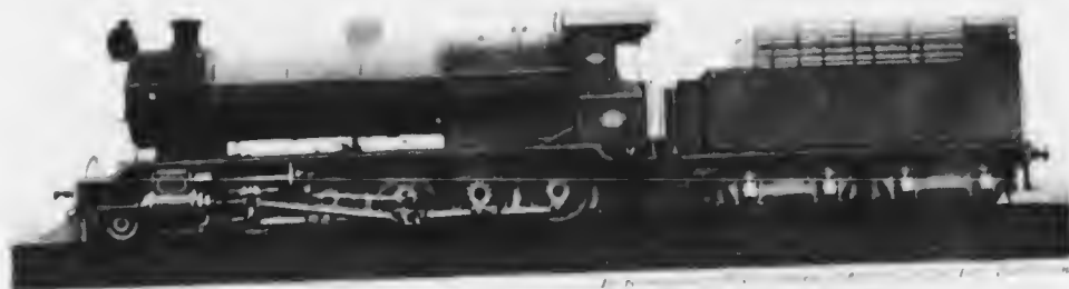
DECAPOD BUILT FOR THE ARGENTINE GREAT WESTERN RAILWAY The line is of 5 feet 6 inches gauge. In working order this locomotive weighs 135 tons complete.
