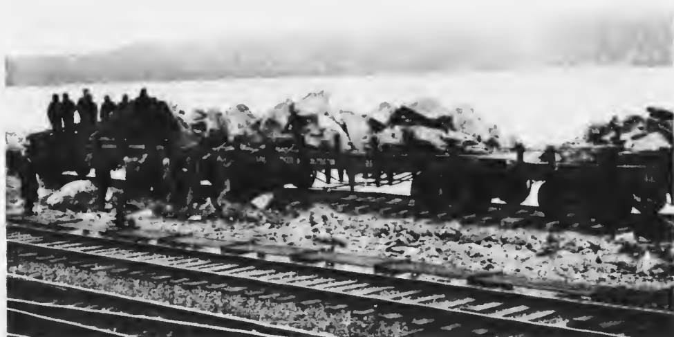
THE LIDGERWOOD UNLOADER DUMPING ROCK FROM A TRAIN. Showing plough and hauling rope.
