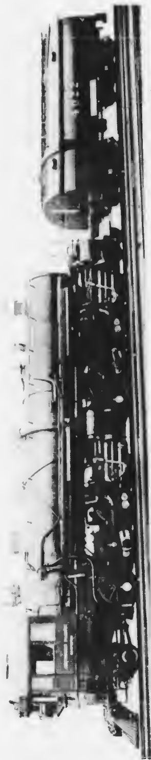
2882 MAMMOTH OIL-BURNING MALLETS ARTICULATED FREIGHT LOCOMOTIVE ON THE SOUTHERN PACIFIC RAILWAY. The cylindrical tender, carrying 10,000 gallons of water and 3,200 gallons of oil, is attached to the chimney end of the engine, while a driving cab is provided on the footplate. In running order the locomotive with tender weighs 306 (U.S.) tons.
