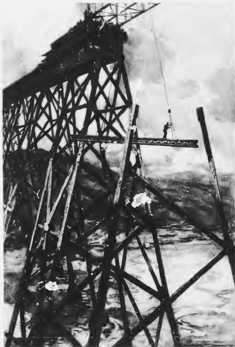
SETTING THE STEEL FOR THE BATTLE RIVER VIADUCT OF THE GRAND TERRITORY PACIFIC RAILWAY.
