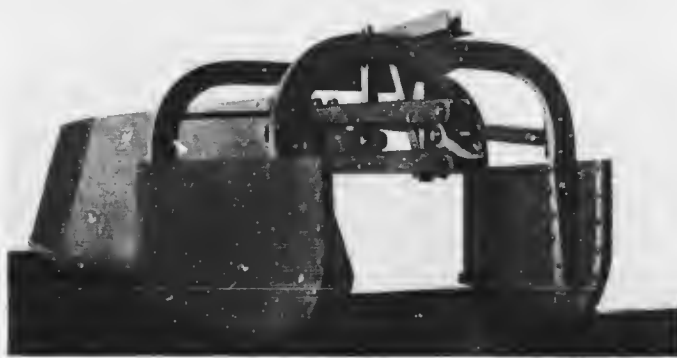
THE BUCYRUS BALLAST DISCHARGING PLOUGH For emptying the contents of the wagons equally on each side.
