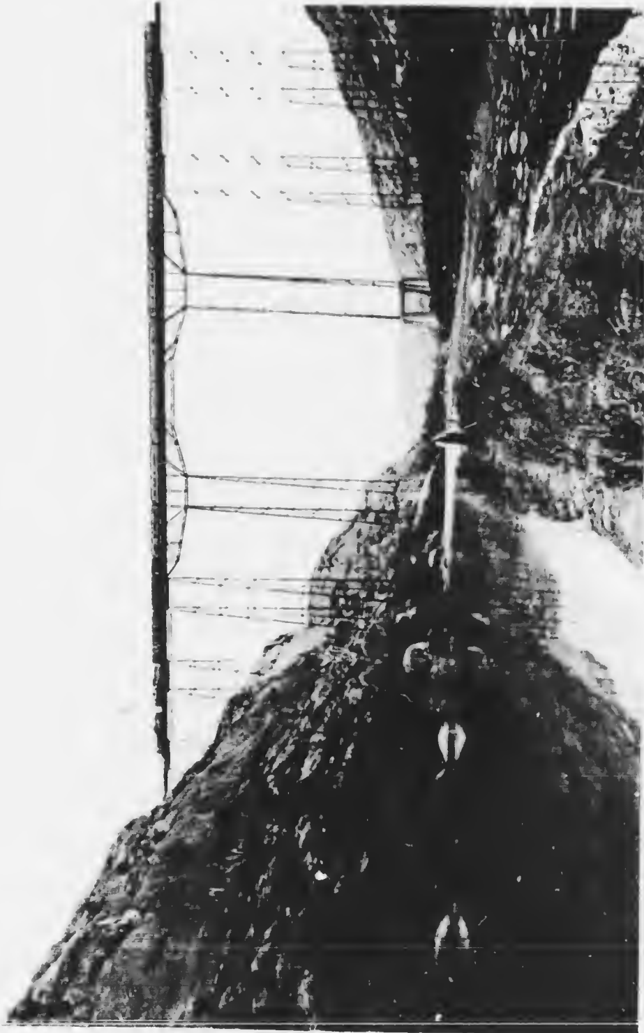
THE RAILS OF THE PECOS HIGH BRIDGE ON THE SOUTHERN PACIFIC RAILWAY, 219 MILES WEST OF SAN ANTONIO ARE 321 FEET ABOVE WATER LINE; THE CANTILEVER SPAN IS 155 FEET IN LENGTH.
