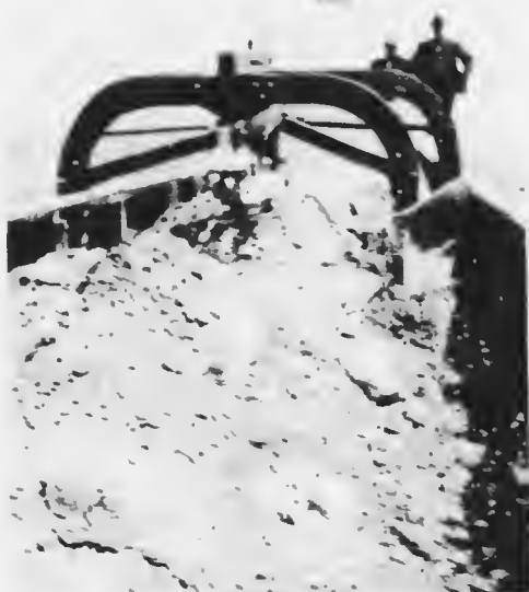
THE BUCYRUS DISCHARGING PLOUGH AT WORK. It is pulled by means of a cable from the extreme rear to the front of the train.
