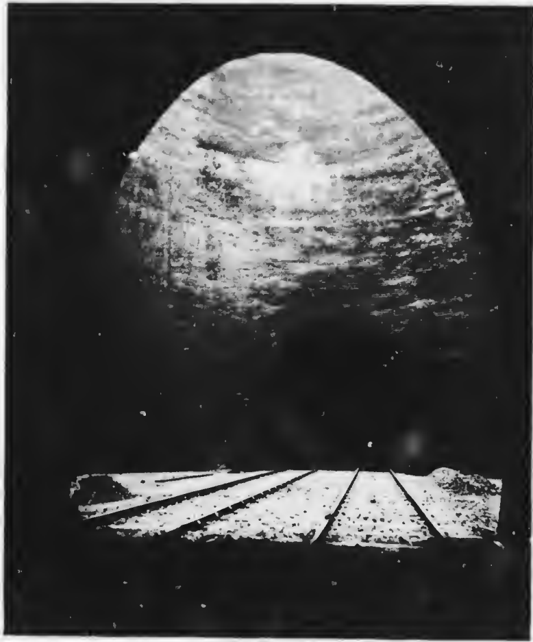
THE MAIN SHAFT IN THE KILSBY TUNNEL.
