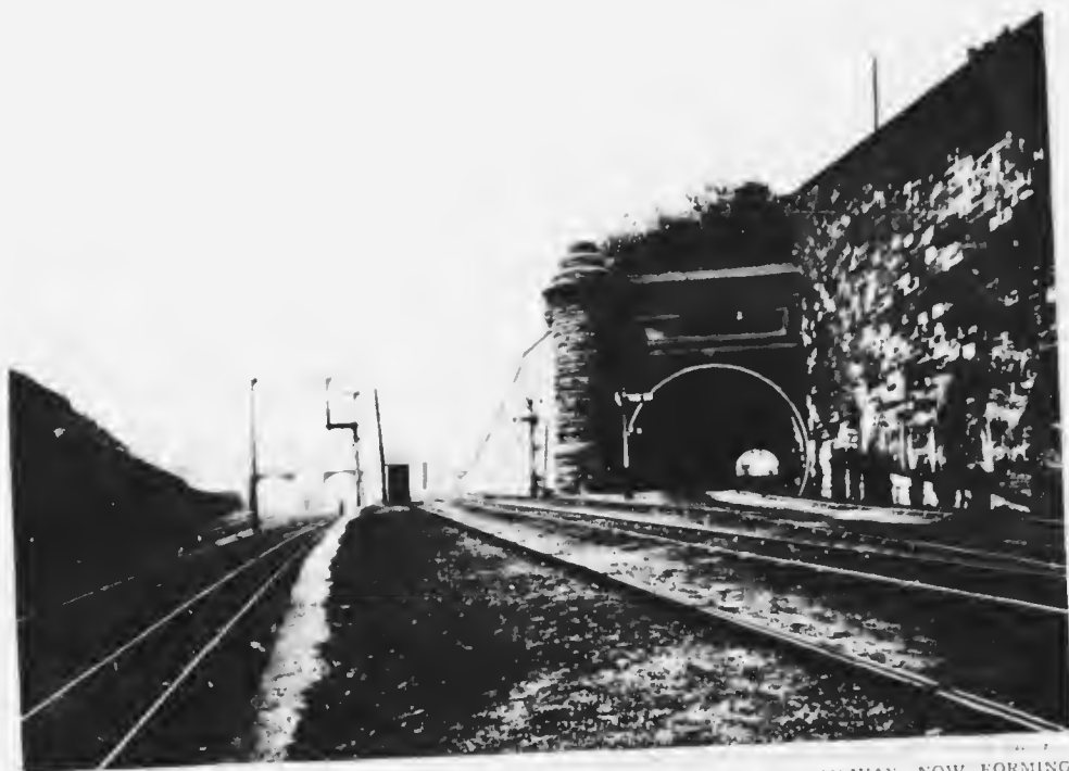
THE FAMOUS OLIVE CUTTING ON THE LIVERPOOL AND MANCHESTER RAILWAY, NOW FORMING PART OF THE LONDON AND NORTH WESTERN SYSTEM
