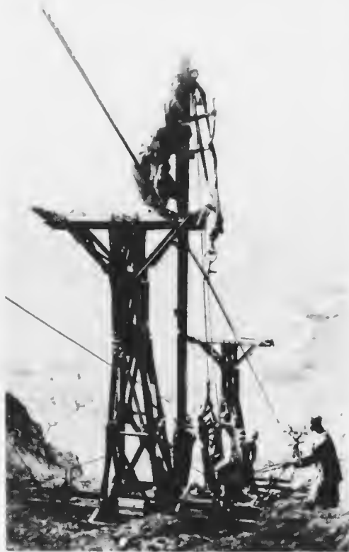
LIFTING THE CABLES UPON THE SUPPORTS.
