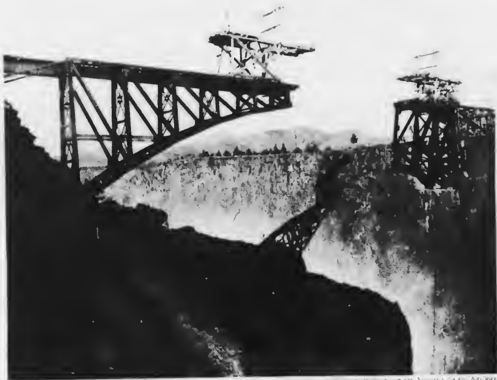
BUILDING THE ARCH SPAN OF THE CROOKED RIVER BRIDGE FROM BOTH SIDES OF THE CANYON SIMULTANEOUSLY, SHOWING THE TWO TRAVELLERS.
