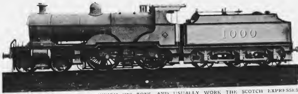
THE "1000" COMPOUND CLASS WEIGH 105.8 TONS, AND USUALLY WORK THE SCOTCH EXPRESSES BETWEEN LONDON AND LEEDS.
