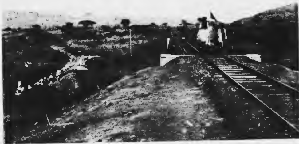
A BIG LOOP ON THE UGANDA RAILWAY TO OVERCOME A SUDDEN STEEP ASCENT.
