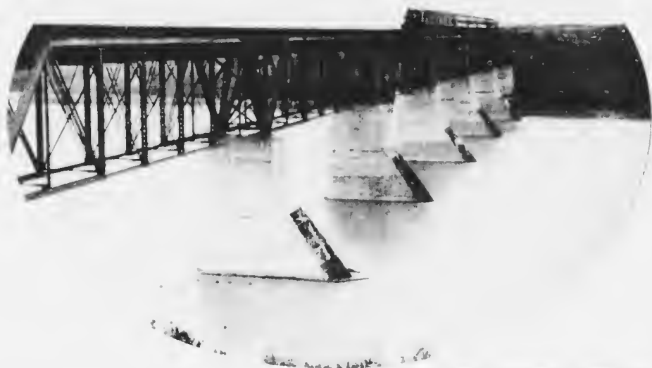
TYPICAL BRIDGE PROVIDED FOR THE CROSSING OF THE WIDE WESTERN CANADIAN RIVERS.
