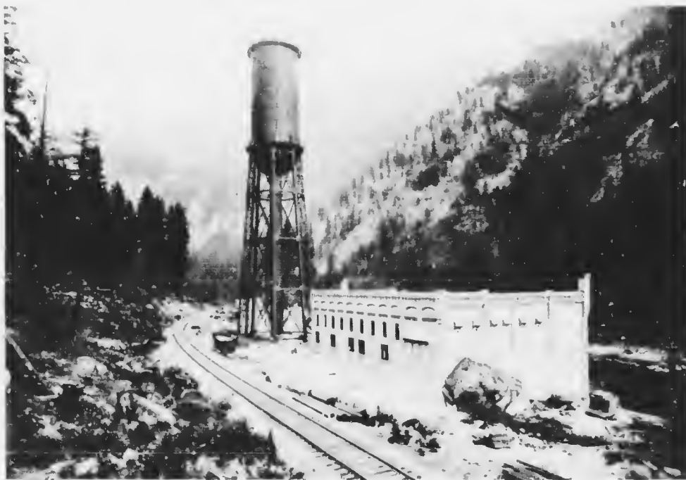
THE POWER-HOUSE IN THE TUMWATER CANYON.
