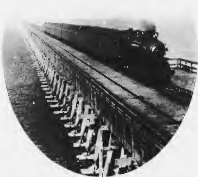
THE TIMBER TRESTLE FORMING THE "CUT-OFF" ACROSS GREAT SALT LAKE.
