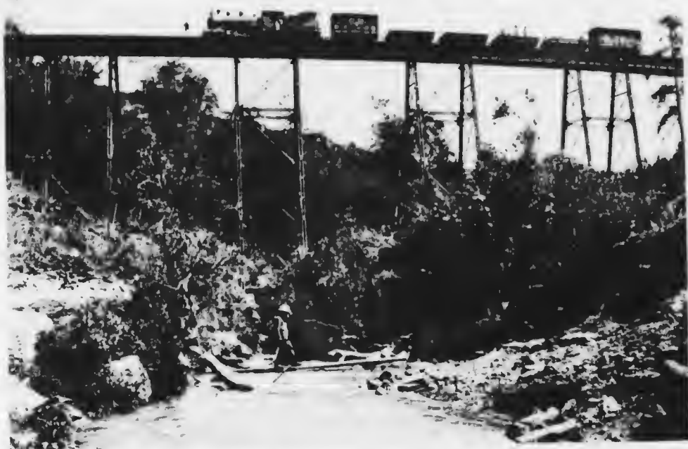
A STEEL TREESTLE BRIDGE ON THE UGANDA RAILWAY
