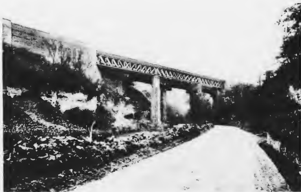
MILLER'S DALE VIADUCTS, 1905.
