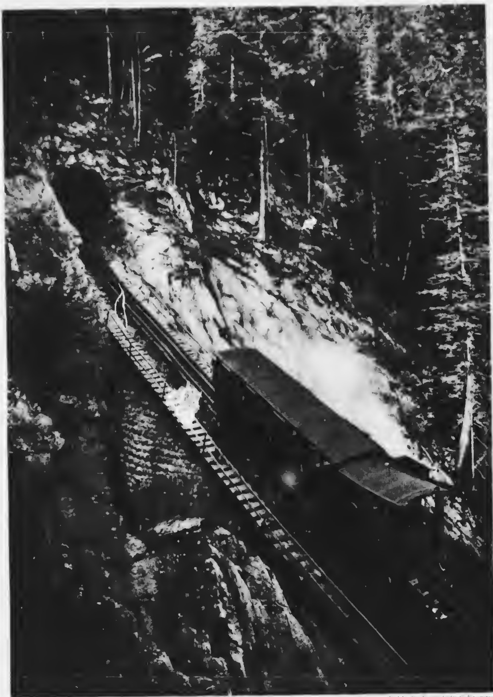
THE STIFFEST BANK ON THE PILATUS RAILWAY.
