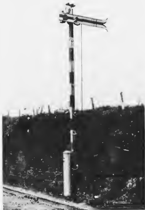
A DISTANT SIGNAL ON THE DANISH STATE RAILWAY, FITTED WITH THE AGA FLASHING LIGHT.
