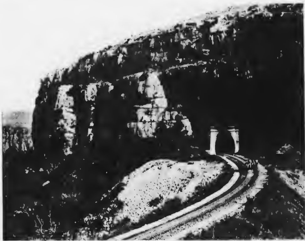
WATERVAL BOVEN TUNNEL ON THE DEVIATION LINE, TRANSVAAL.
