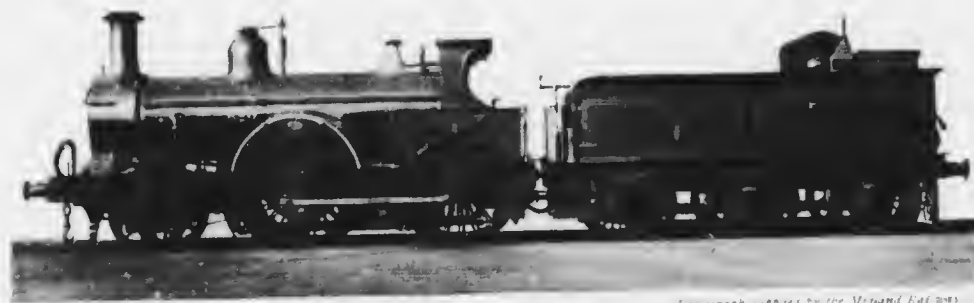
LOCOMOTIVE NO. 820: REMARKABLE FOR ITS HEAVY OUTSIDE FRAME.
