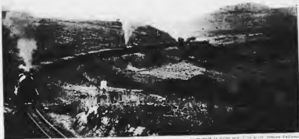
HOW THE HEAVY COAL TRAINS ARE LIFTED OVER THE 1 IN 30 BANKS UPON THE NATAL SECTIONS OF THE SOUTH AFRICAN RAILWAYS. Three locomotives, one at each end and another in the centre, are used.
