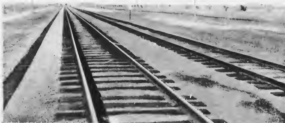
ROAD-BED BALLASTED WITH SHERMAN GRAVEL.
