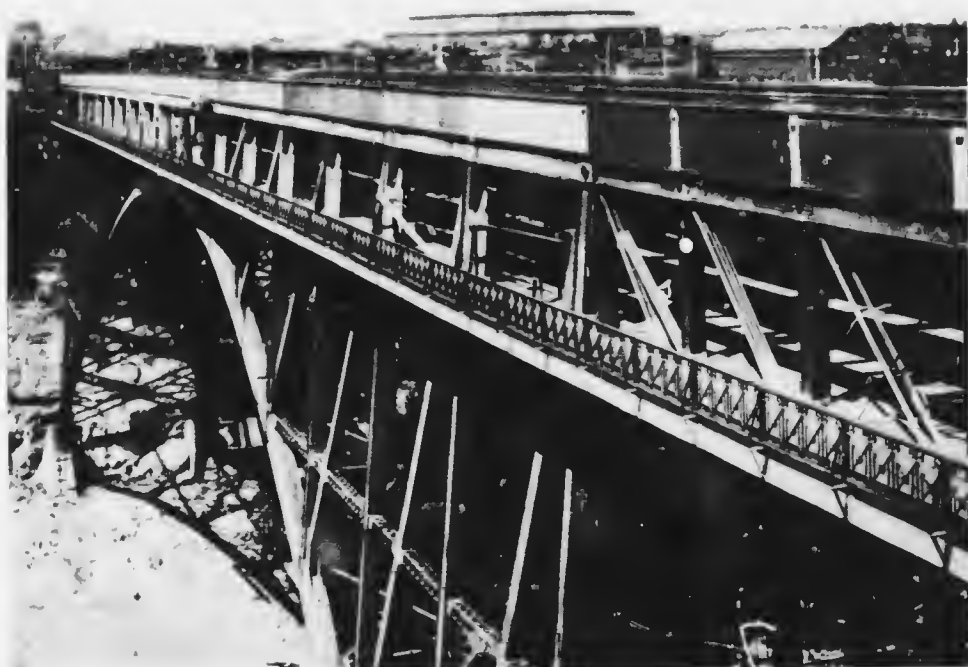
VIEW OF THE NIAGARA SPAN BRIDGE AFTER THE REMOVAL OF THE SUSPENSION BRIDGE. Showing top railway deck and lower deck for public use
