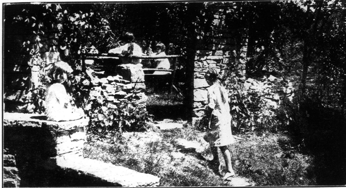
NOT IN THE BACKWOODS, BUT A SCENE NEAR THE CITY LIMITS — A PRETTY BUNGALOW NEAR HIGH PARK, AT THE HEAD OF GRENADIER POND.
