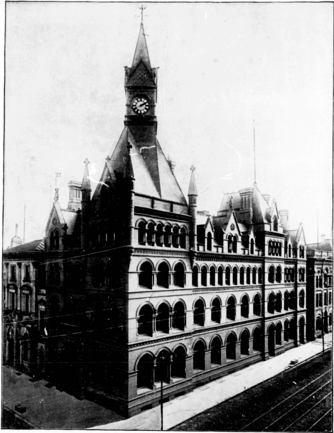
Canada Life Assurance Co. Building.
