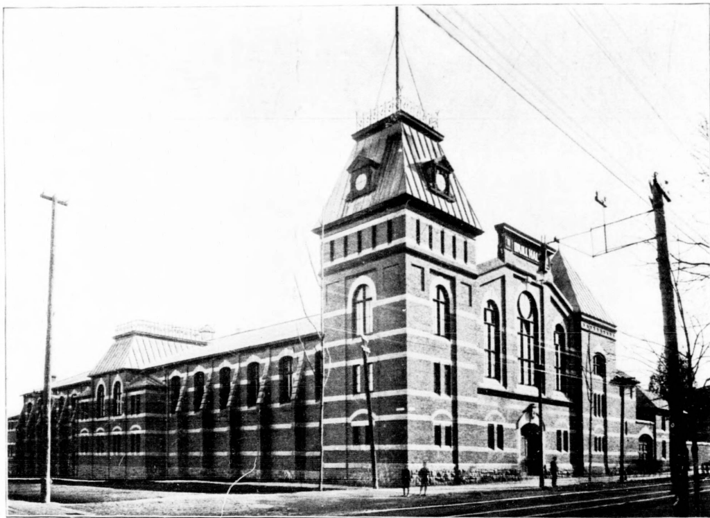
The Drill Hall.
