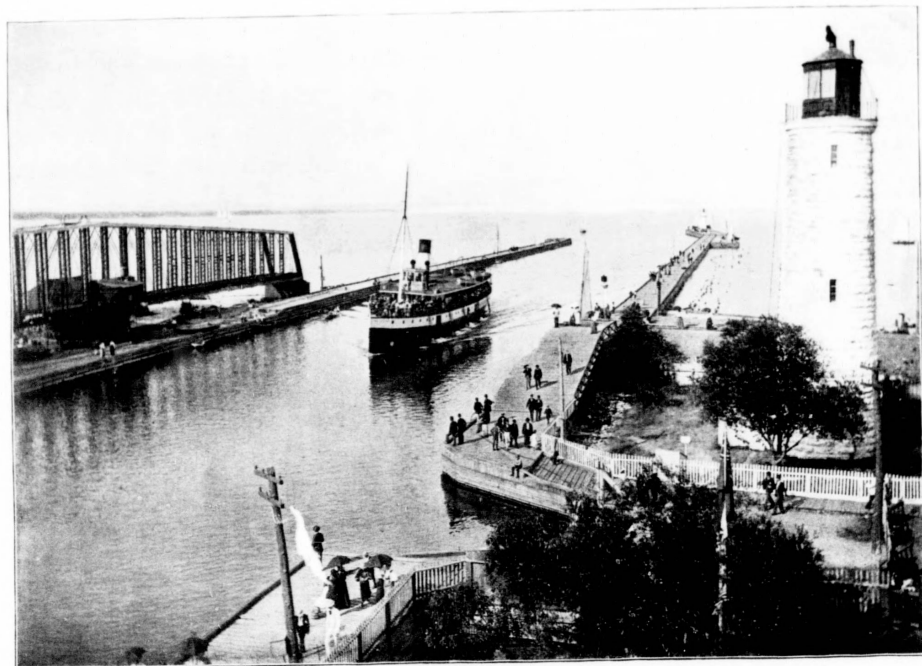
Lighthouse and Drawbridge
