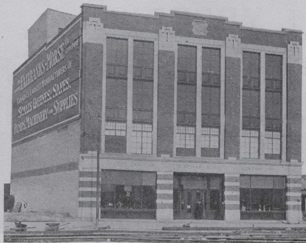
The New Fairbank-Morse Building, Saskatoon
