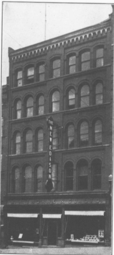
The new Edison sign at W. H. Thorne Co.'s, St. John, N.B., in the day time as at night. The size of the letters is 16 in. x 12 in. The total length of the sign is 24 ft. The background is dark brown, with a gold and green border with red inserts. Its appearance at night is very attractive."
