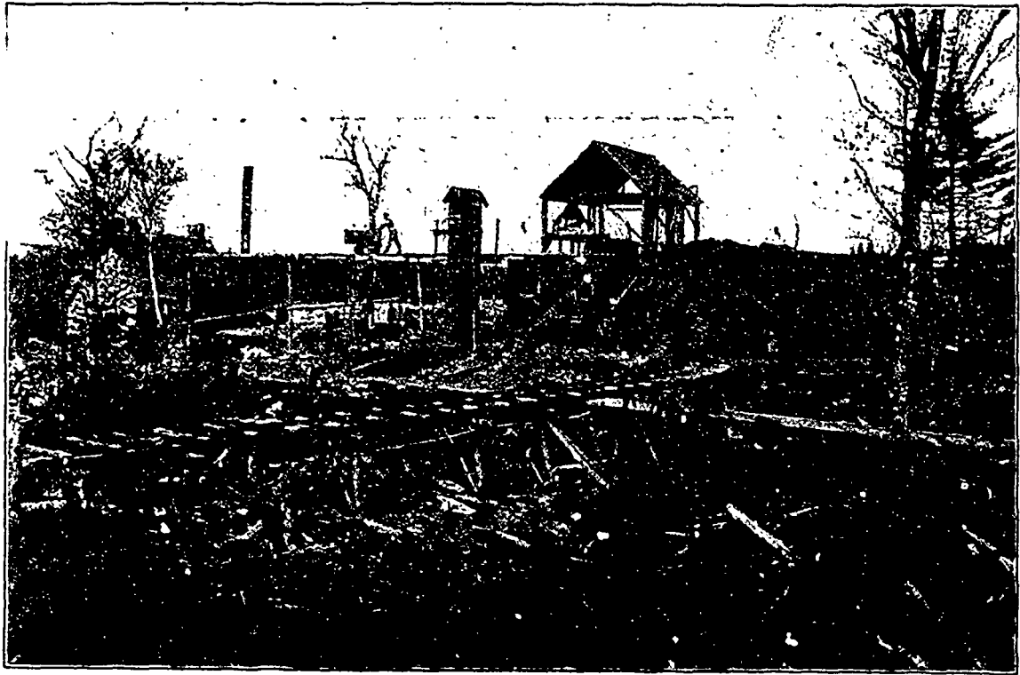
MODSTOCK GOLD MINING CO.—Main Shaft and Mill, Forest Hill, Stormont District, Nova Scotia.
