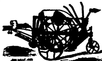
ELEVATOR DITCHING MACHINE FOR UNDERDRAINING.
