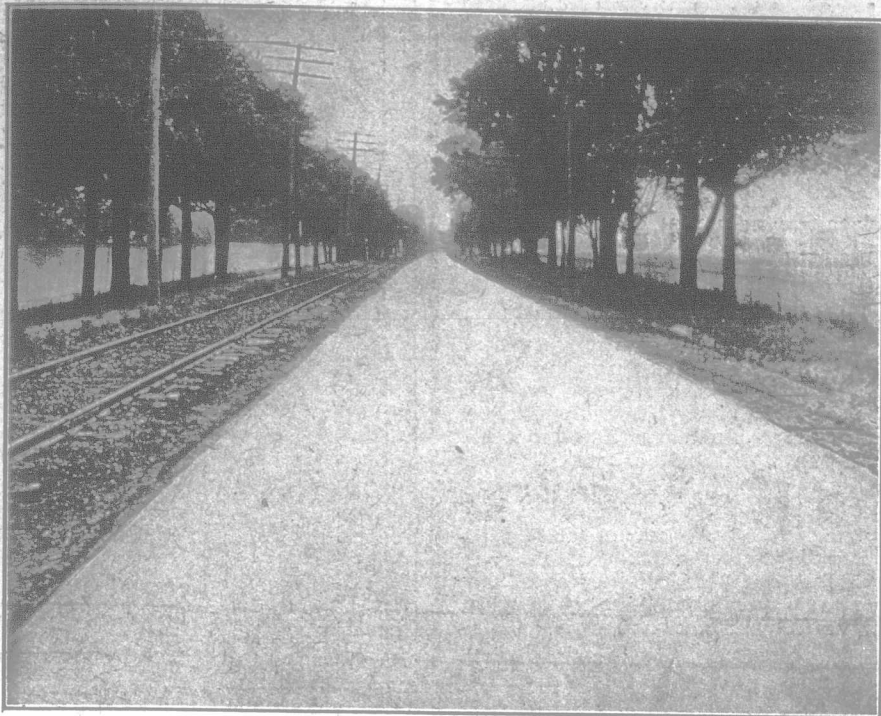
No ruts on this or any other concrete road
