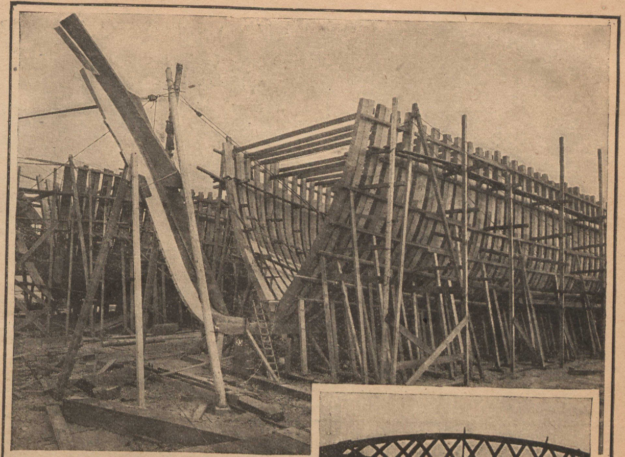
Ribs of a wooden ship, built at North Vancouver, in a land of limitless wood.
