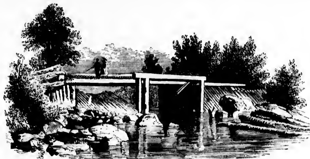
LUMBER DAM AND SLUICE.
