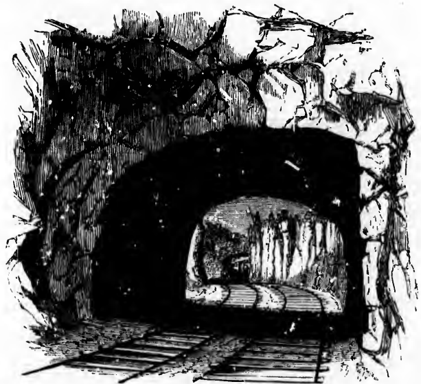
TUNNEL AT FLAT POINT.
