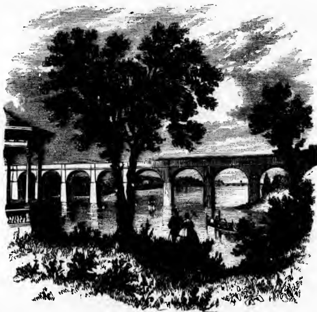
THE HIGH BRIDGE.*
