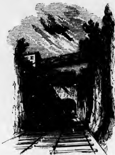
NEW HAMBURG TUNNEL.
