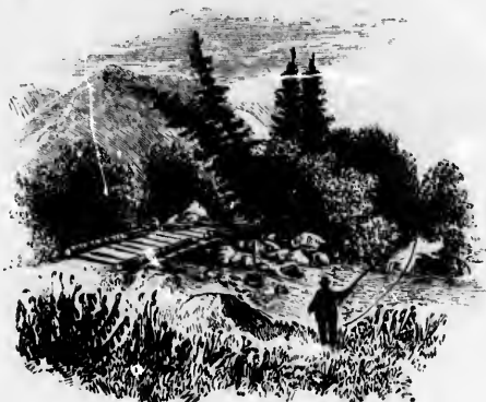
FIRST BRIDGE OVER THE HUDSON.
