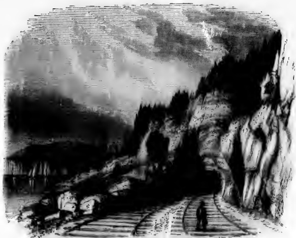
TUNNEL AT ANTHONY'S NOSE.
