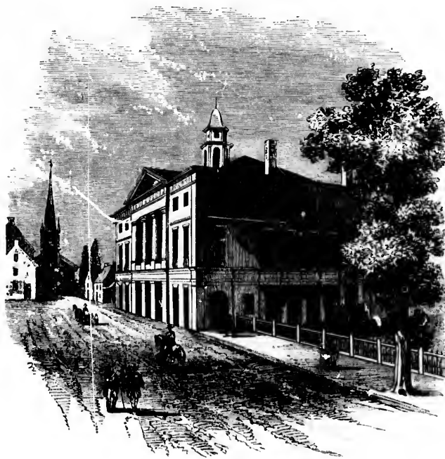
OLD FEDERAL HALL.
